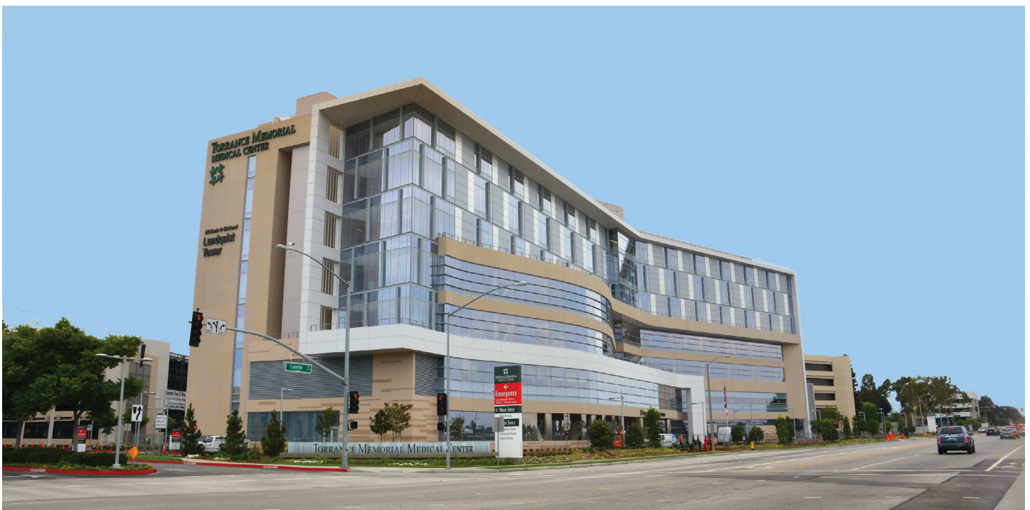
Melanie and Richard Lundquist Tower, Torrance Memorial Medical Center
